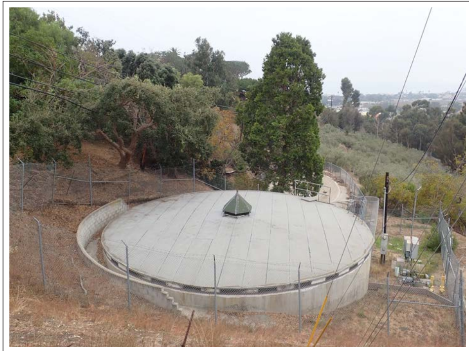
Photo 1. View of existing Serra water tank. Taken facing south
