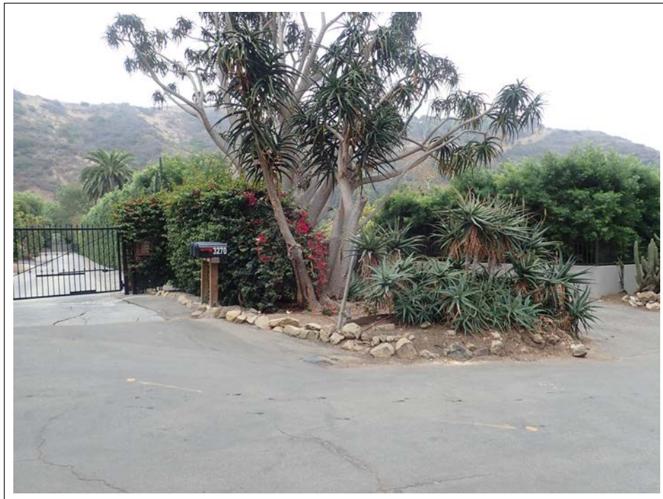
Photo 3. Intersection of Palm Canyon Lane and Serra Road. Location of one of the Pressure Regulating Stations. Taken facing north.
