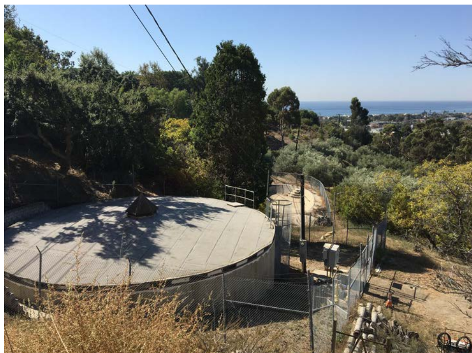
View 2 – View of the existing Serra Tank facing south.
